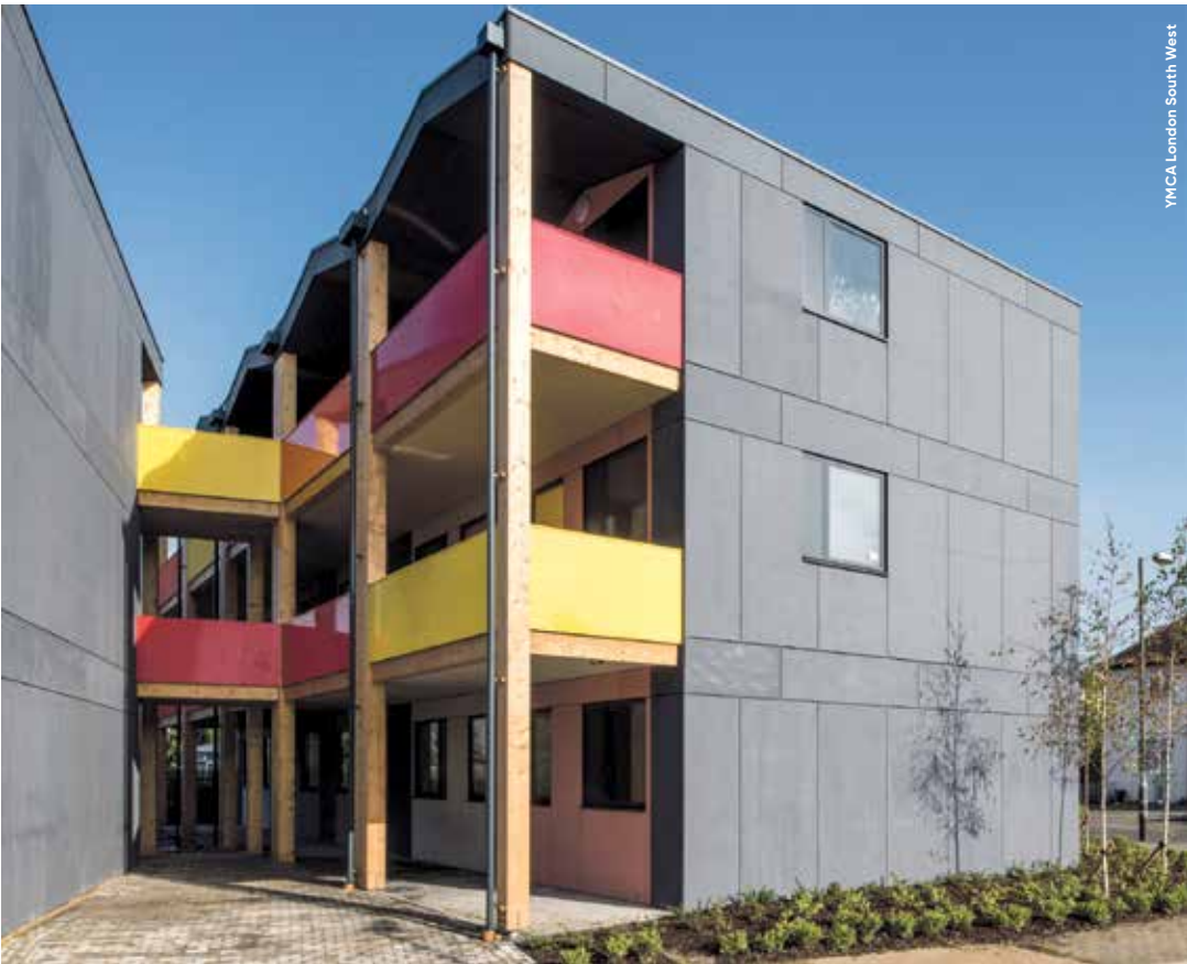
Y:Cube units made for the YMCA in Mitcham, south London; the development is made up of 36 modular, studio-like apartments 280sq ft in floor area and constructed off-site in a factory
